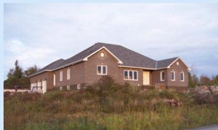
October 1 – the start of the project
