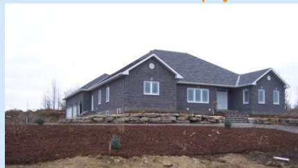
November 10 – the completed project
